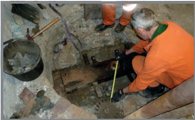
Positioning the new bearing and greasing system.
