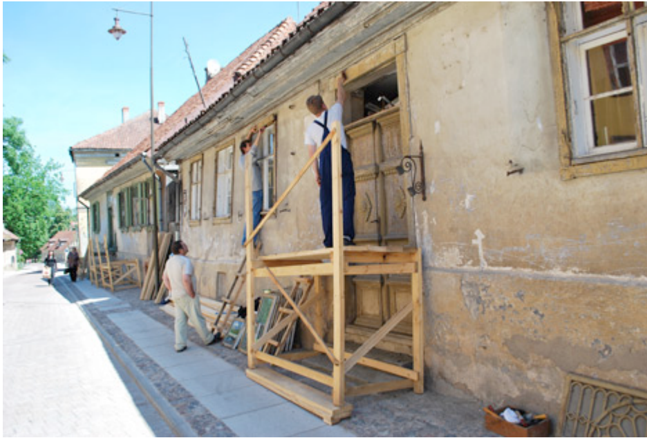
Works in Kalna street.
