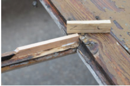
Restoration of glazing bar.
