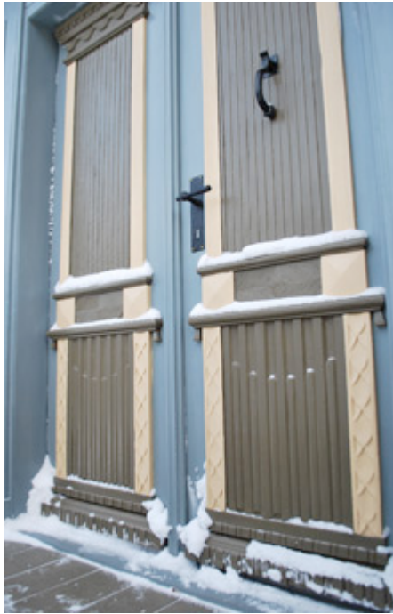
The newly restored door in Kalna street, 15, Kuldiga.
