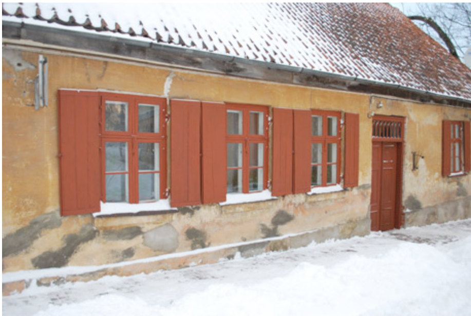
Baznica gate 28, Restored windows, window shutters and doors.
