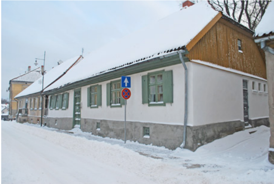
Kalna gate 13, Restored door, windows, window shutters and wall.
